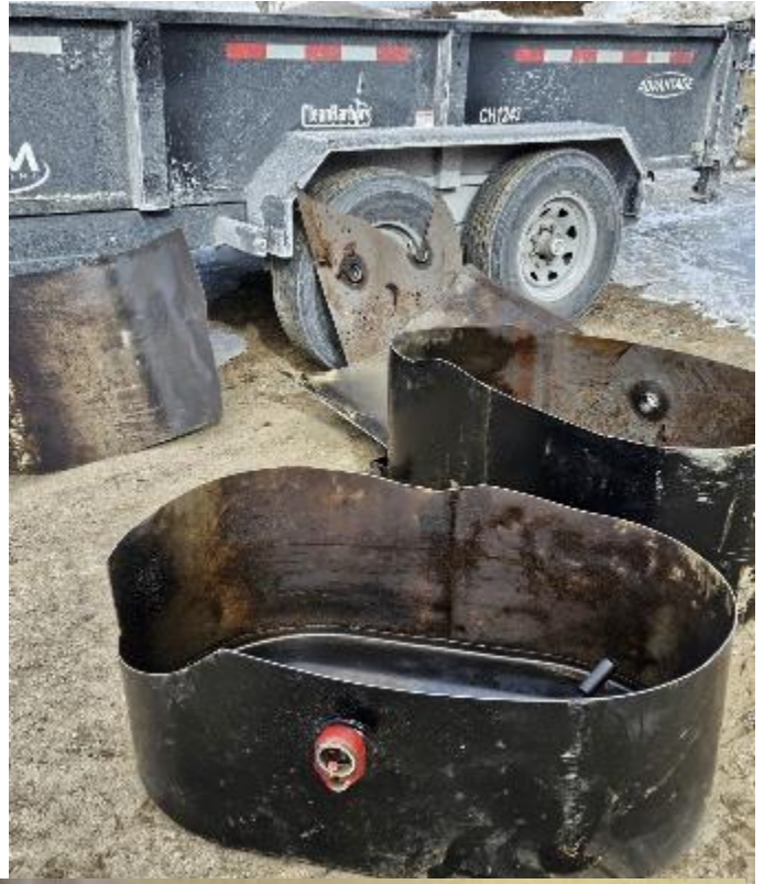
Oil tanks cleaned, then cut up, and removed from crawl space area. Thank God they were removed before the fire! Fire pictures on next page.
