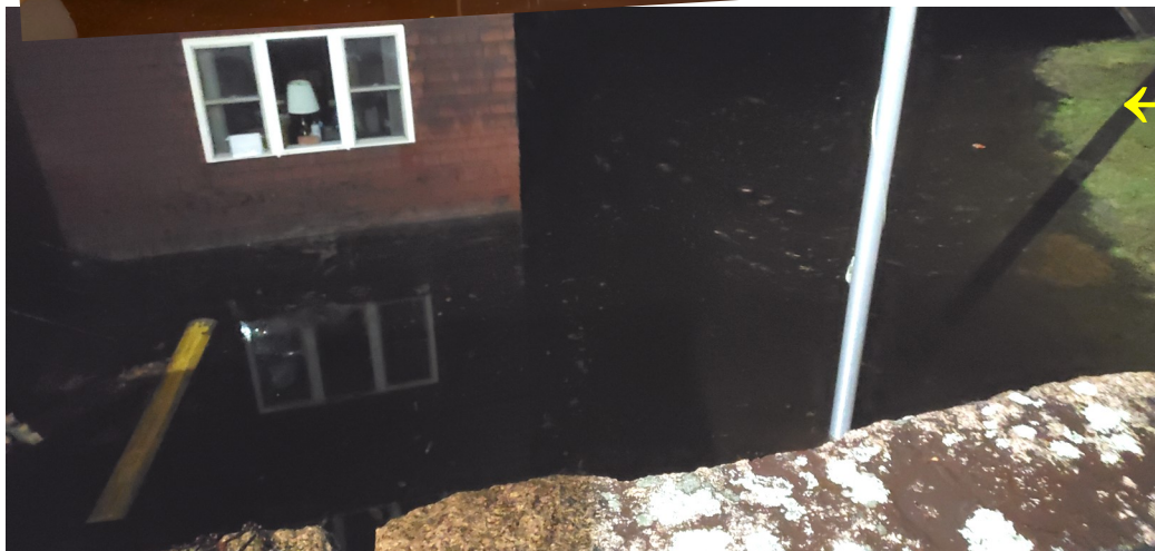
Looking down from handicap ramp
